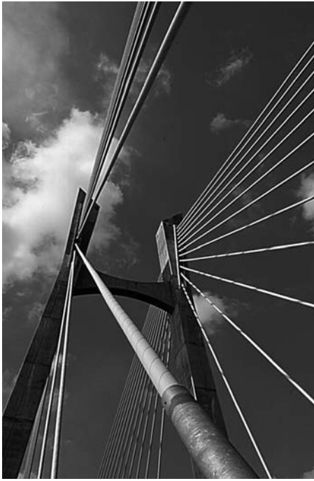
Figure 49. A duct of the Beaucaire Bridge with the helical filets.
