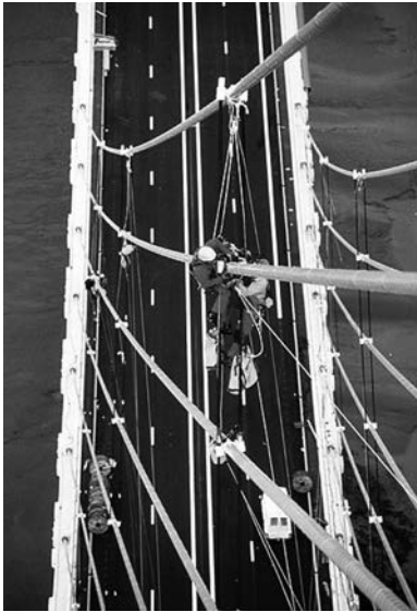
Figure 55. Installation of the aiguilles at the Normandie Bridge.
