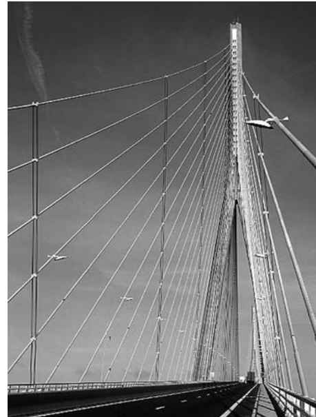
Figure 56. Duct and cross-cables at the Normandie Bridge (photo courtesy of Freyssinet).
