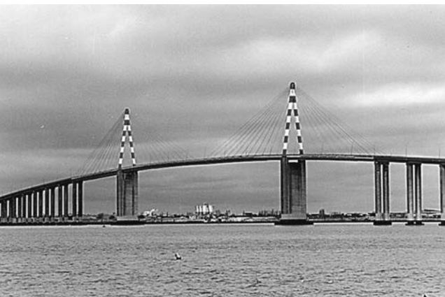
Figure 3. The Saint-Nazaire Bridge.
