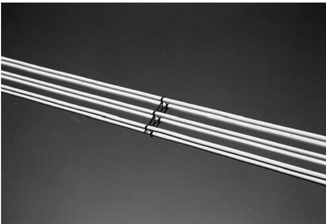
Figure 27. Six backstays at the Erasmus Bridge attached to avoid wake effects.
