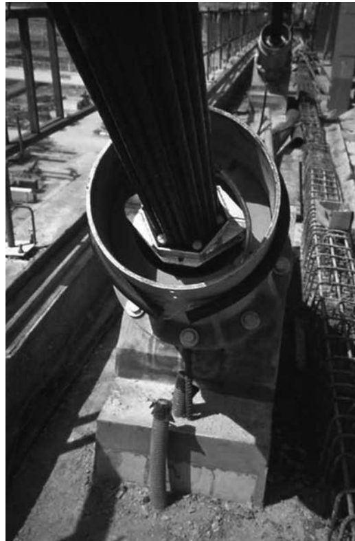
Figure 46. A damper at the Vasco de Gama Bridge (photo courtesy of Freyssinet).
