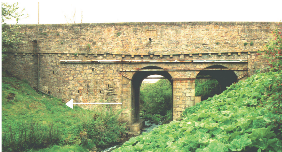
Fig. 5. Elevation of North Middleton masonry arch bridge.
