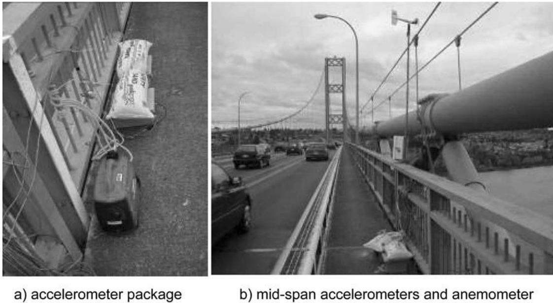
Figure 7. Field measurement set up on the Existing Tacoma Bridge.
