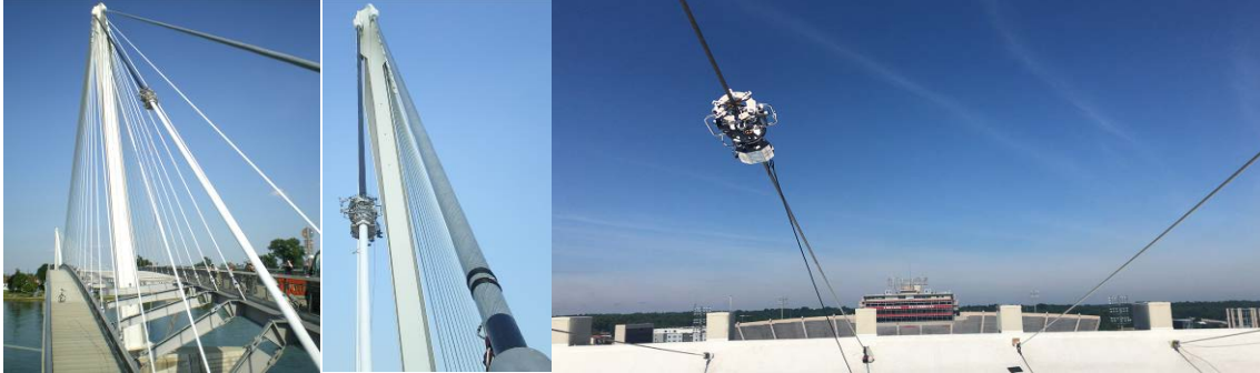
Figure 4. Fully automated wrapping of ATIS Cableskin ® . Left: Passerelle Des Deux Rives, France / Germany, 76 stay cables, 2500 m 2 , 2008. Right: Assembly Hall Indiana University, US, 8 supporting cables, 2019.
