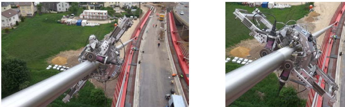
Figure 11. Fully automated polishing robot travelling along a stay cable of Mersch Red Bridge, Luxembourg, 2016. Left: Device traveling downwards while polishing the stainless-steel surface. Right: Detail. Polishing module rotated about 90° compared to the left image.
