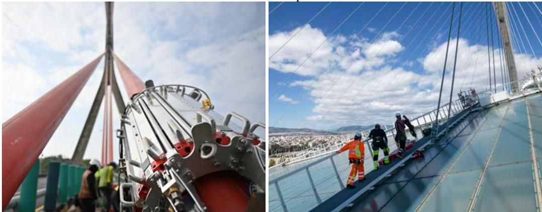
Figure 7. Application of the R315 MRT device designed by DYWIDAG at Kao Ping Bridge -Taiwan (left), application of the R140 MRT device designed by DYWIDAG at Olympic Stadium Athens – Greece (right).
